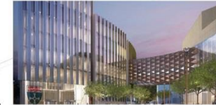
2) Learning & Teaching Centre Completion date: Autumn 2017
