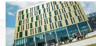
4) The Core Completed: November 2014
