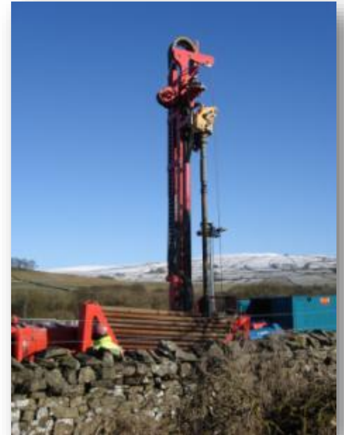
Eastgate 2, Geothermal research well, Durham
