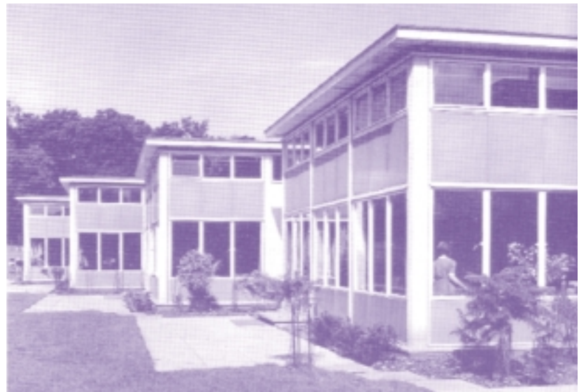
Figure 5 Templewood School, Herts LEA, built 1949–50, showing the steel frame construction (above) and complete (below) (Saint, 1987, p. 80)
