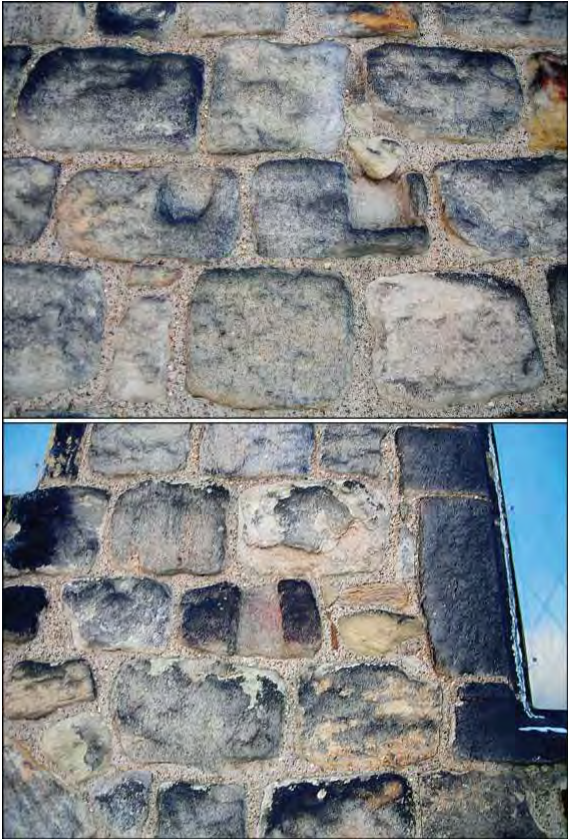
Figure 11: Roman cut mouldings, visible on north external elevation of the Eastern Church at Jarrow.
