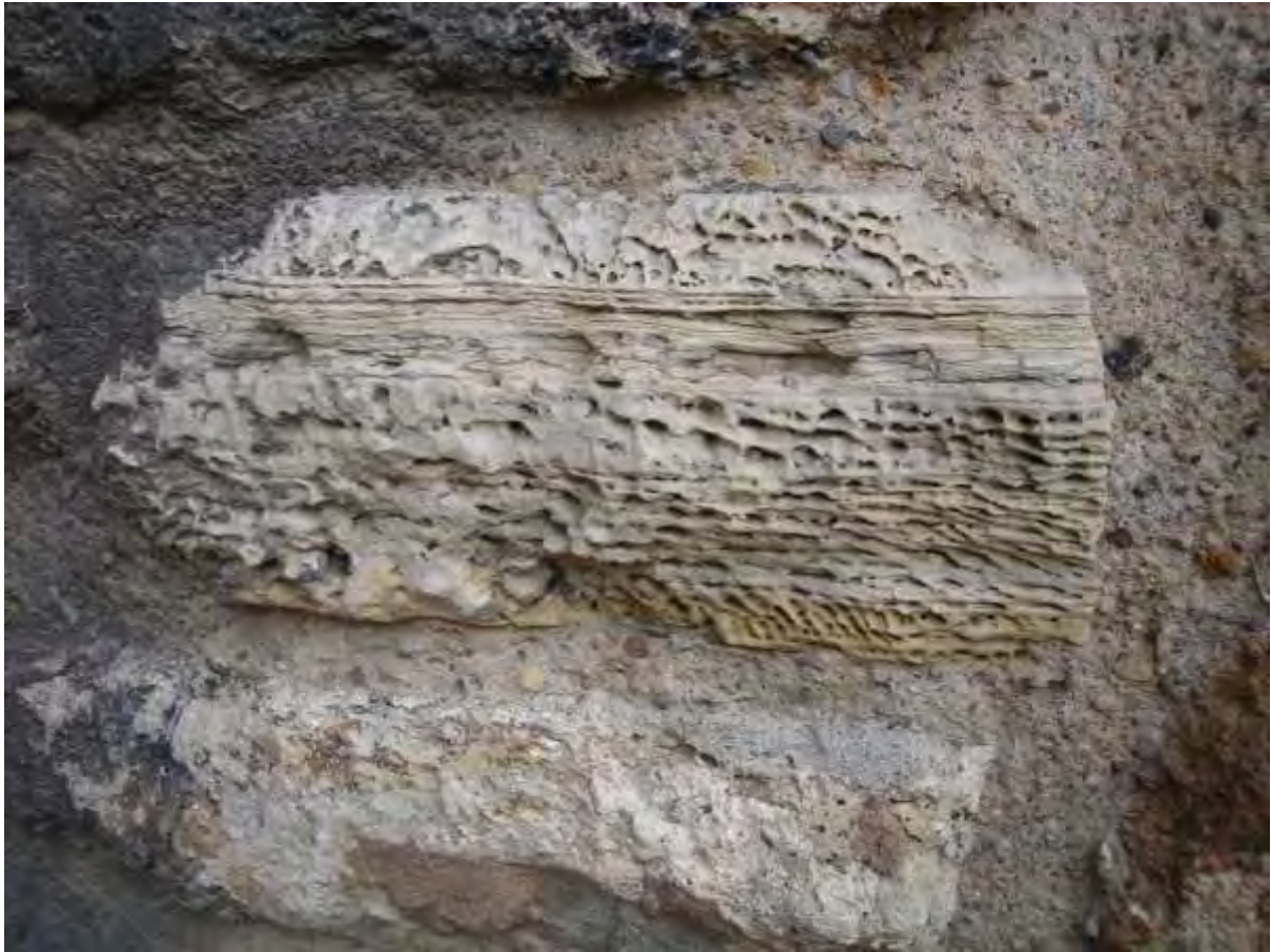
Figure 35c: Sample of cellular structures in Concretionary Limestone, Upper Permian present in the standing fabric at St. Peter's, Wearmouth.
