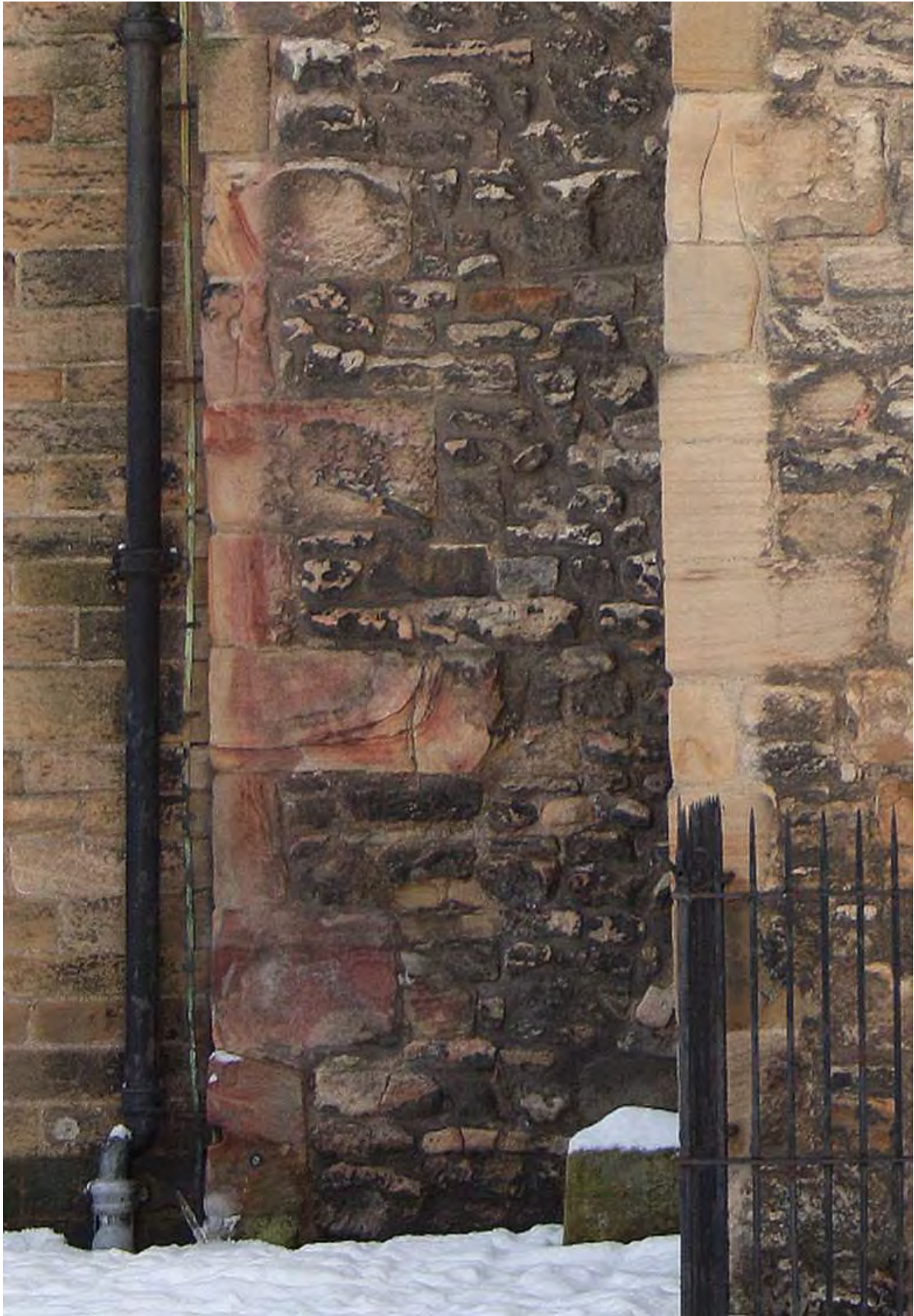
Figure 4: Original quoins at north-west corner of the original nave at St. Peter's, Wearmouth. Note the burned stonework
