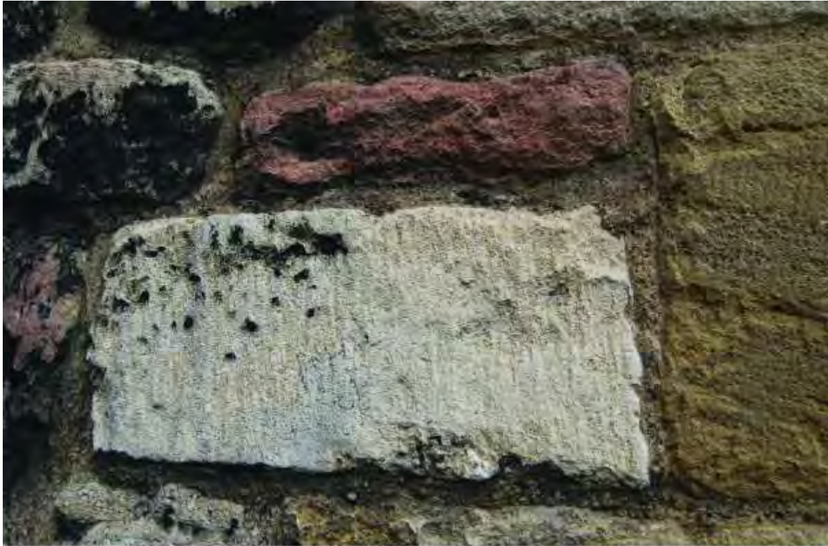
Figure 24: Heddon-on-the-Wall: squared rubble walling. Note the c. 30 cm lift dimension.
