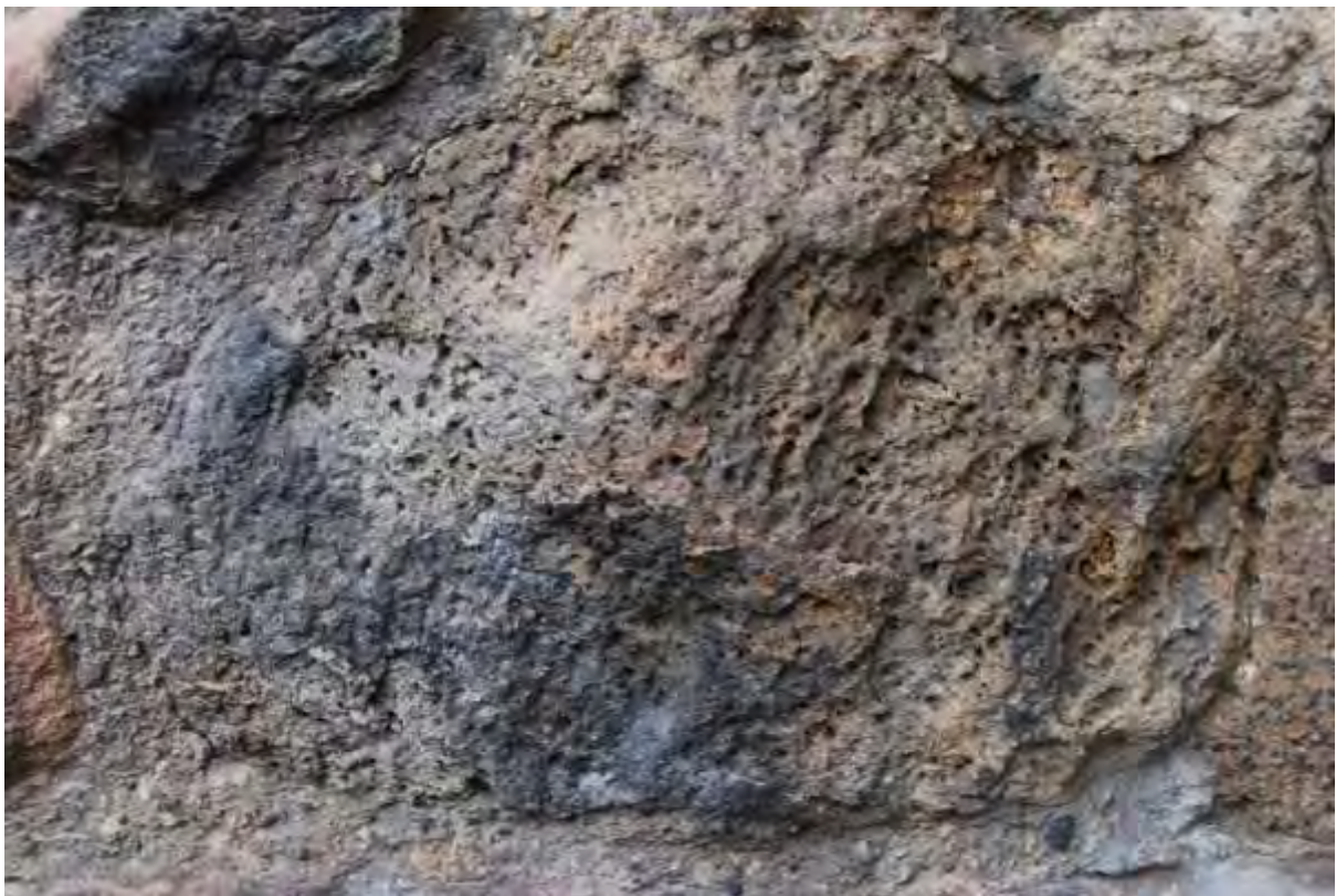
Figure 35a: Sample of cellular structures in Concretionary Limestone, Upper Permian present in the standing fabric at St. Peter's, Wearmouth.
