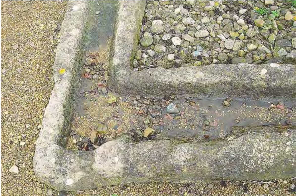
Figure 27a: Drainage culverts at Segedunum, executed from 70 fathom Post Sandstone.
