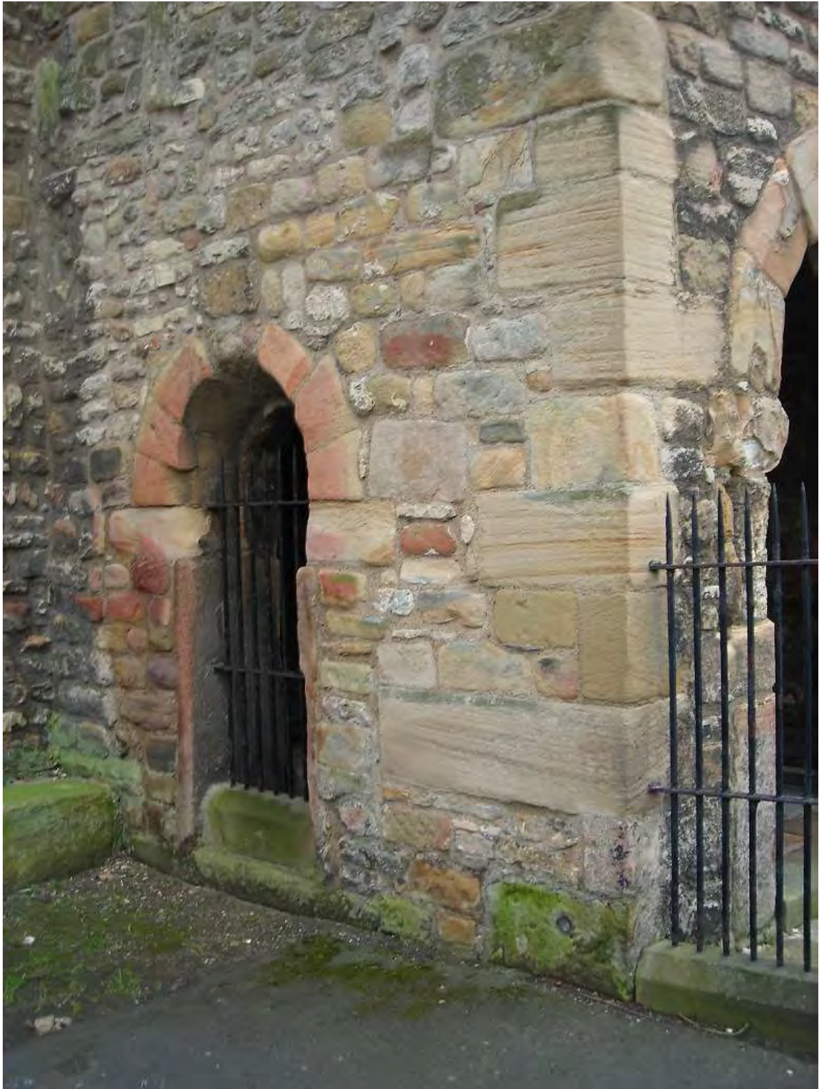
Figure 3a: Entrance on north side of the porch, St. Peter's, Wearmouth. Shows burned ashlar in situ.
