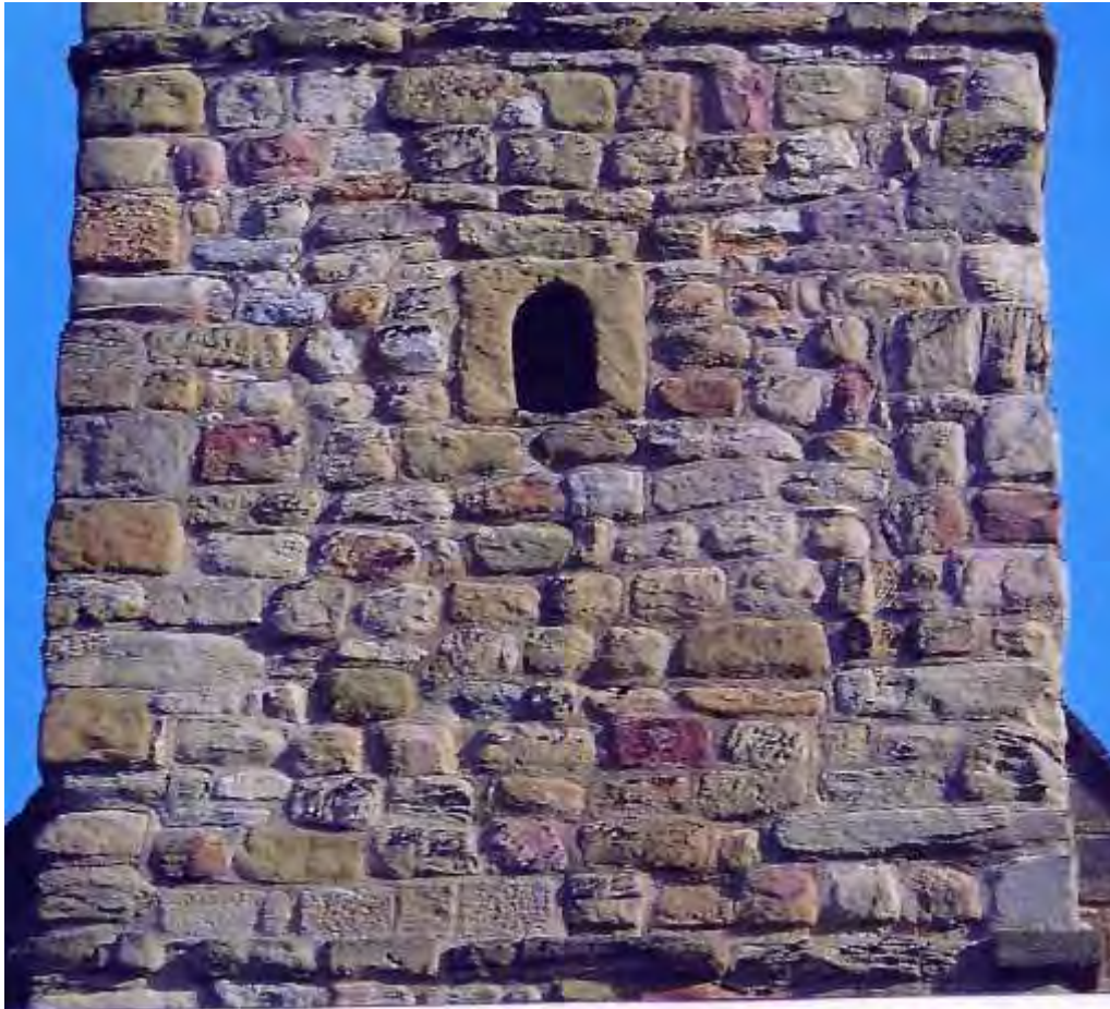
Figure 19: The 11th-century tower at St. Peter's, Wearmouth: not the extensive use of Roman squared stone, largely executed in Wrekenton sandstone.
