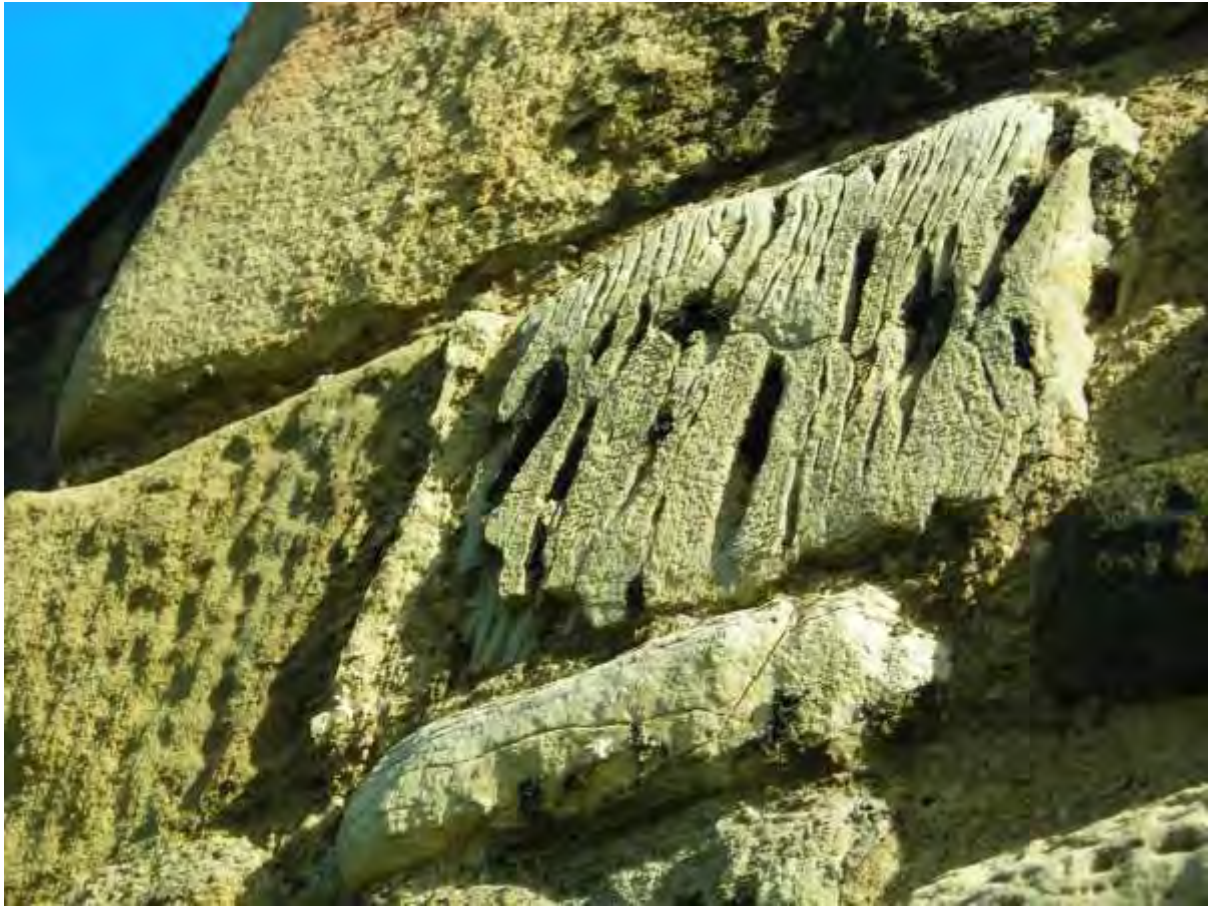
Figure 35b: Sample of cellular structures in Concretionary Limestone, Upper Permian present in the standing fabric at St. Peter's, Wearmouth.
