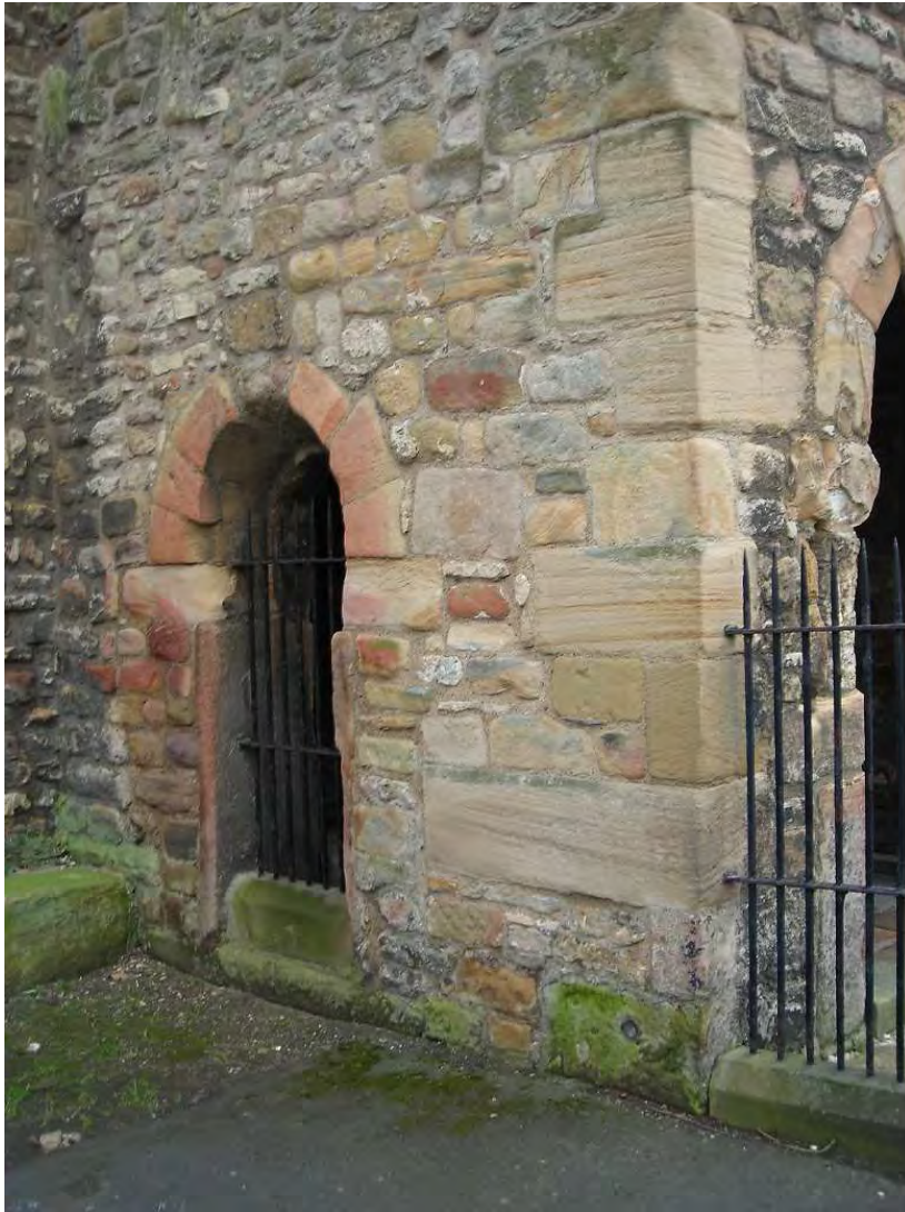
Figure 39: The north doorway of the porch at St. Peter's Church, Wearmouth, showing considerable fire reddening on the stone.
