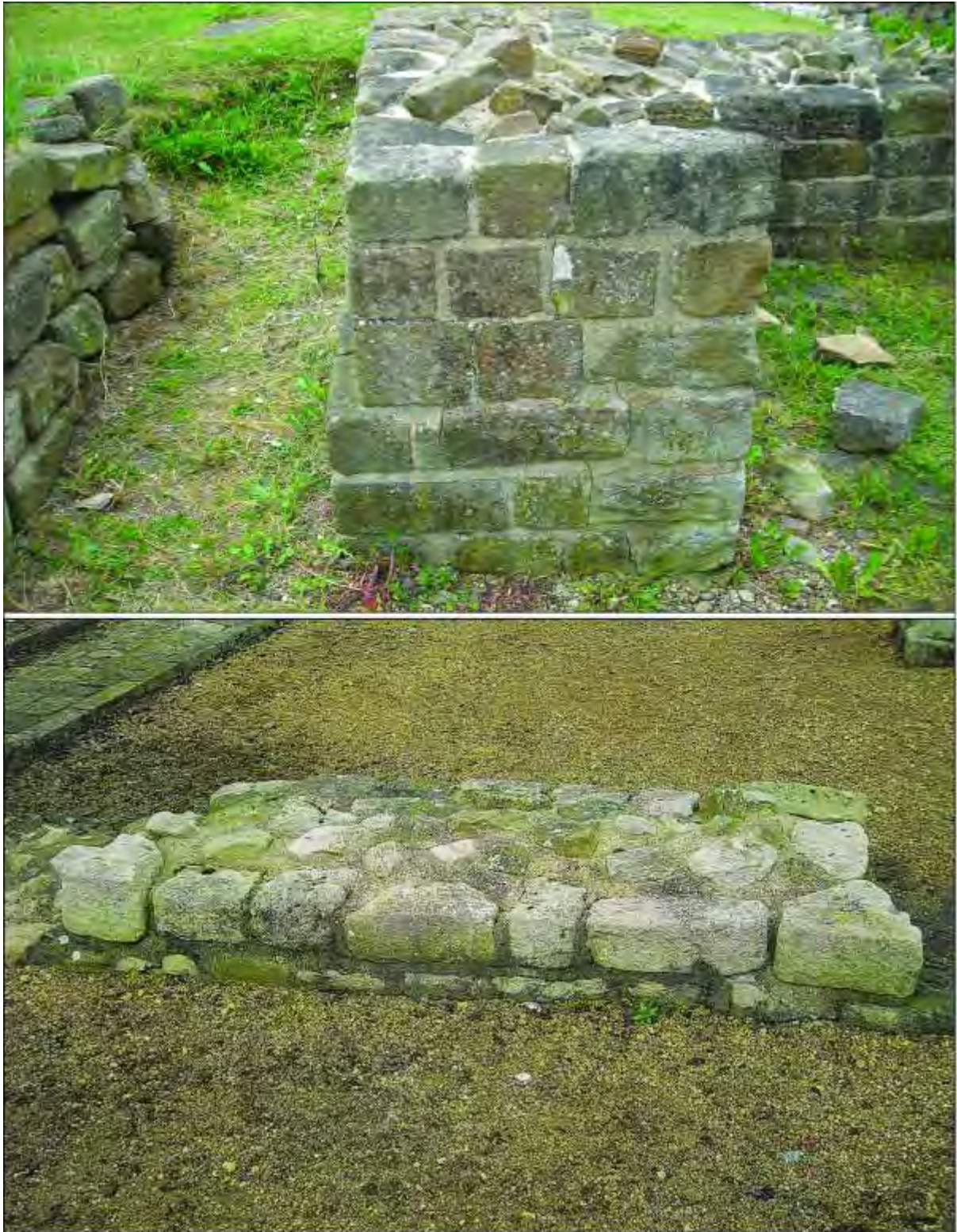
Figure 17: Top: Arbeia: standard 25 x 25 x 25cm squared ashlar executed in Wrekenton Sandstone. Bottom: Segedunum: squared rubble walling executed in Millstone Grit with a lift height of c. 15 cm
