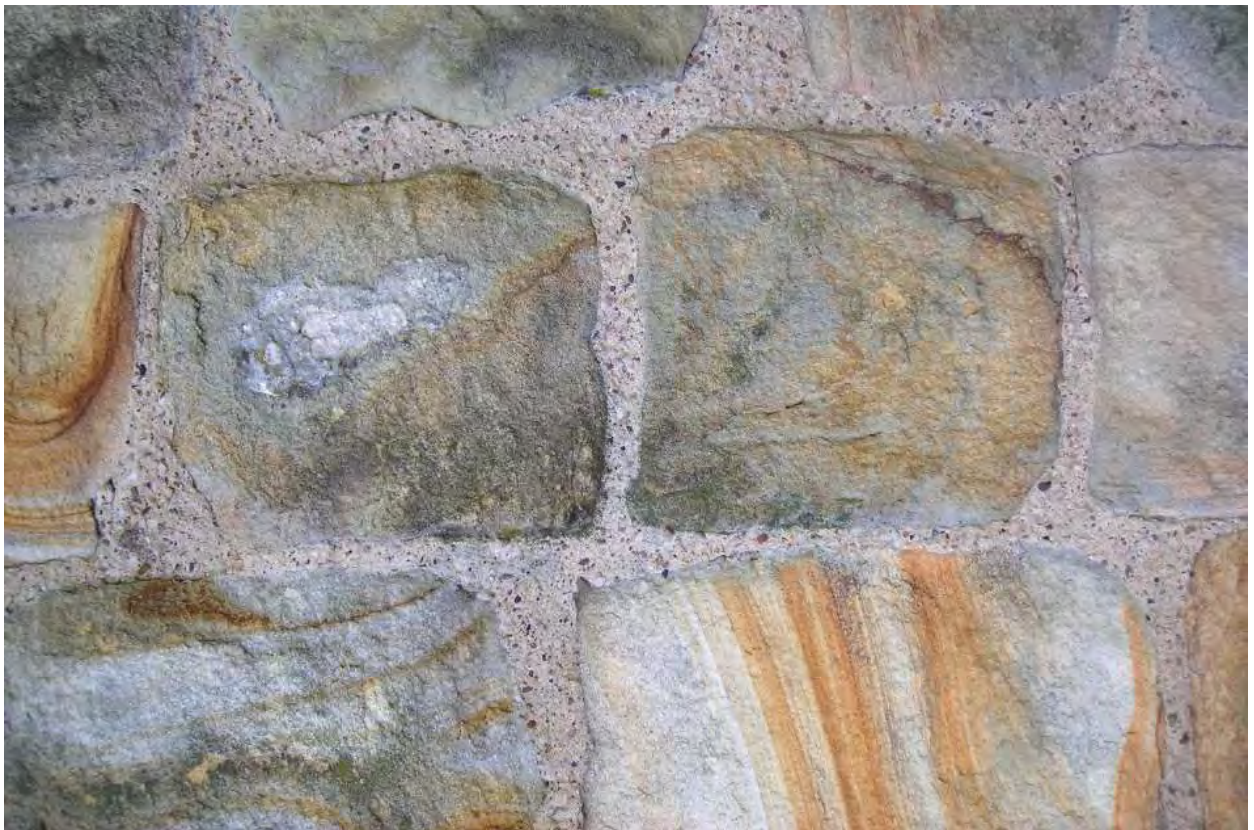
Figure 29: Roman cut stone blocks reused at Jarrow. Exterior, north-west corner of Eastern Church. Stones appear to have been burned prior to their use in the pre-Conquest structure.
