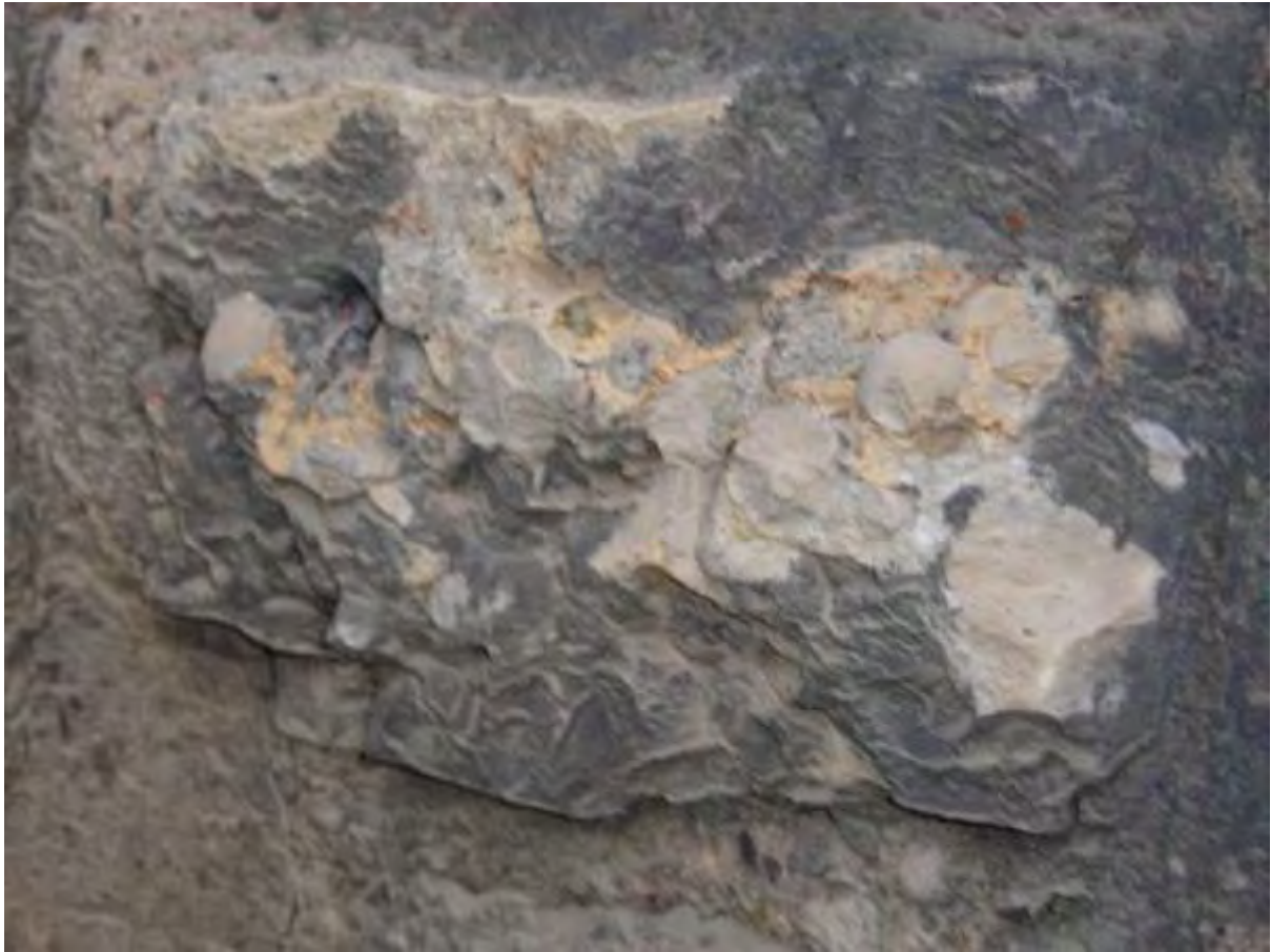
Figure 34a: Types of Permian Roker Dolomite (Lower Magnesian Limestone) present in the standing fabric at St. Peter's, Wearmouth: a) Cannonball Limestone
