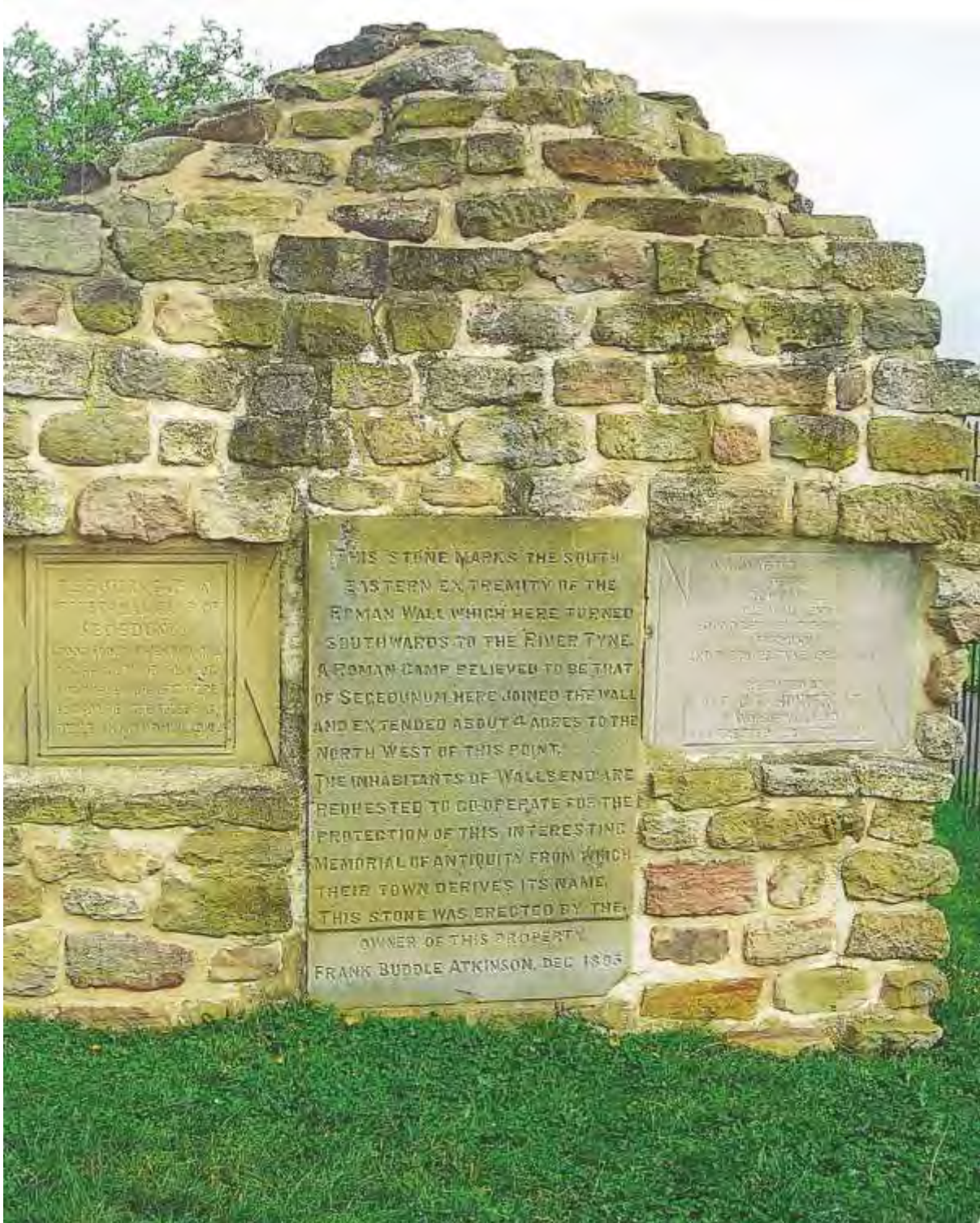
Figure 28: Recently constructed walling supporting 19th and 20th century commemoration slabs. Constructed from Roman squared rubble, probably from Arbeia.
