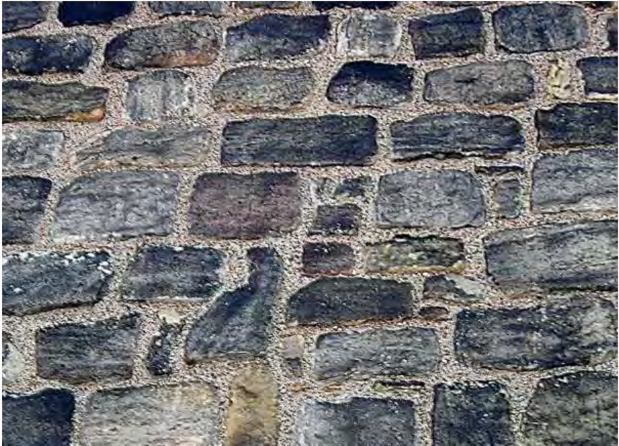
Figure 16: Roman squared building stone – saxa quadrata – west end of the exterior north wall at Jarrow.
