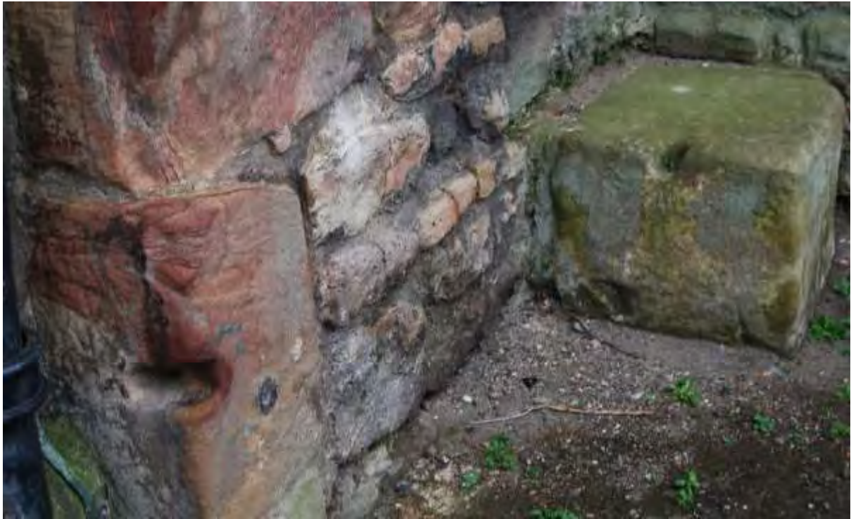
Figure 14: Lewis holes visible in quoin used at the north-west corner of the west external face of the porch at St. Peter's, Wearmouth. The block has been split in two for use in the early medieval building.
