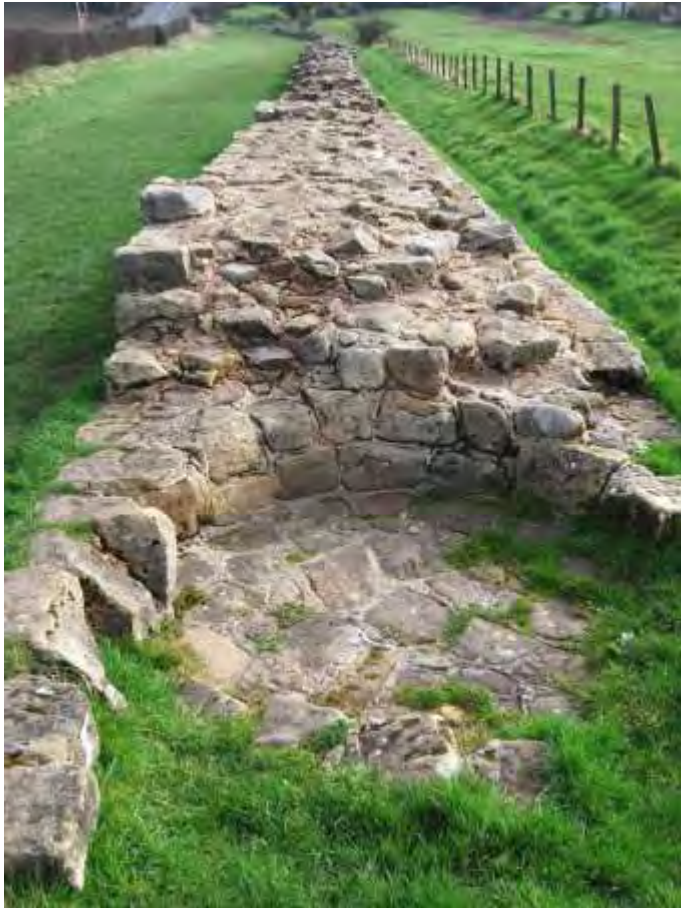
Figure 23: Roman Wall section at Heddon-on-the-Wall, constructed with local Millstone Grit ('Third Grit' Lower Carboniferous; NZ 130668).
