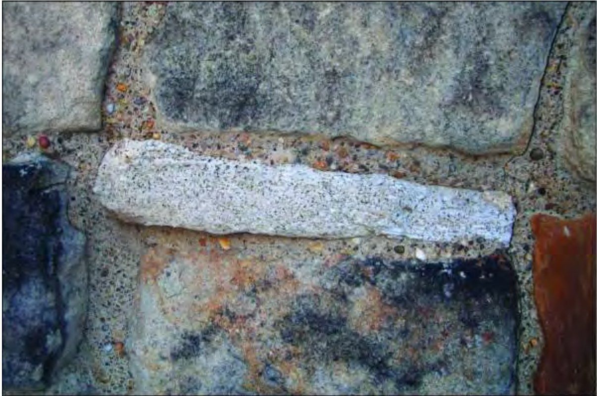
Figure 32: Arbeia: squared rubble walling in Dean Sandstone (Type B). Note the pick shade to the body colour of the stone.
