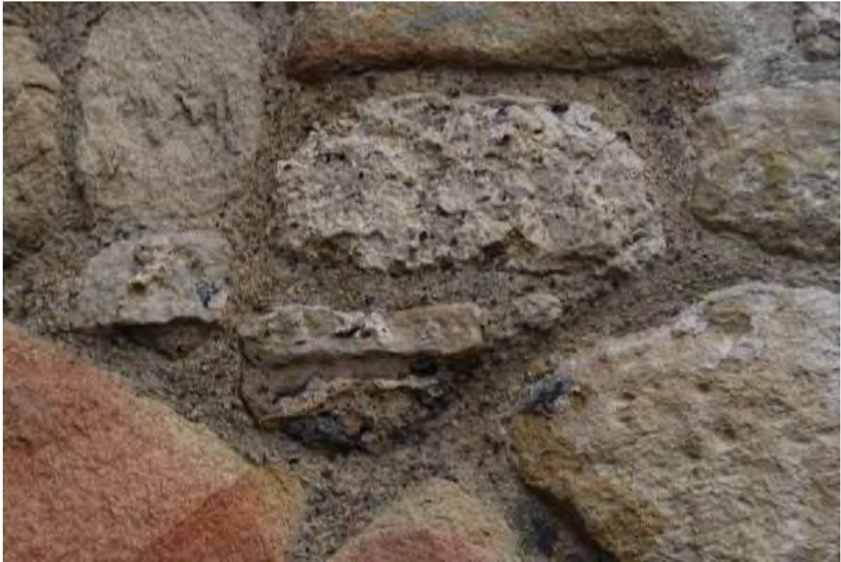
Figure 34b: Types of Permian Roker Dolomite (Lower Magnesian Limestone) present in the standing fabric at St. Peter's , Wearmouth: b) Spherulite Limestone
