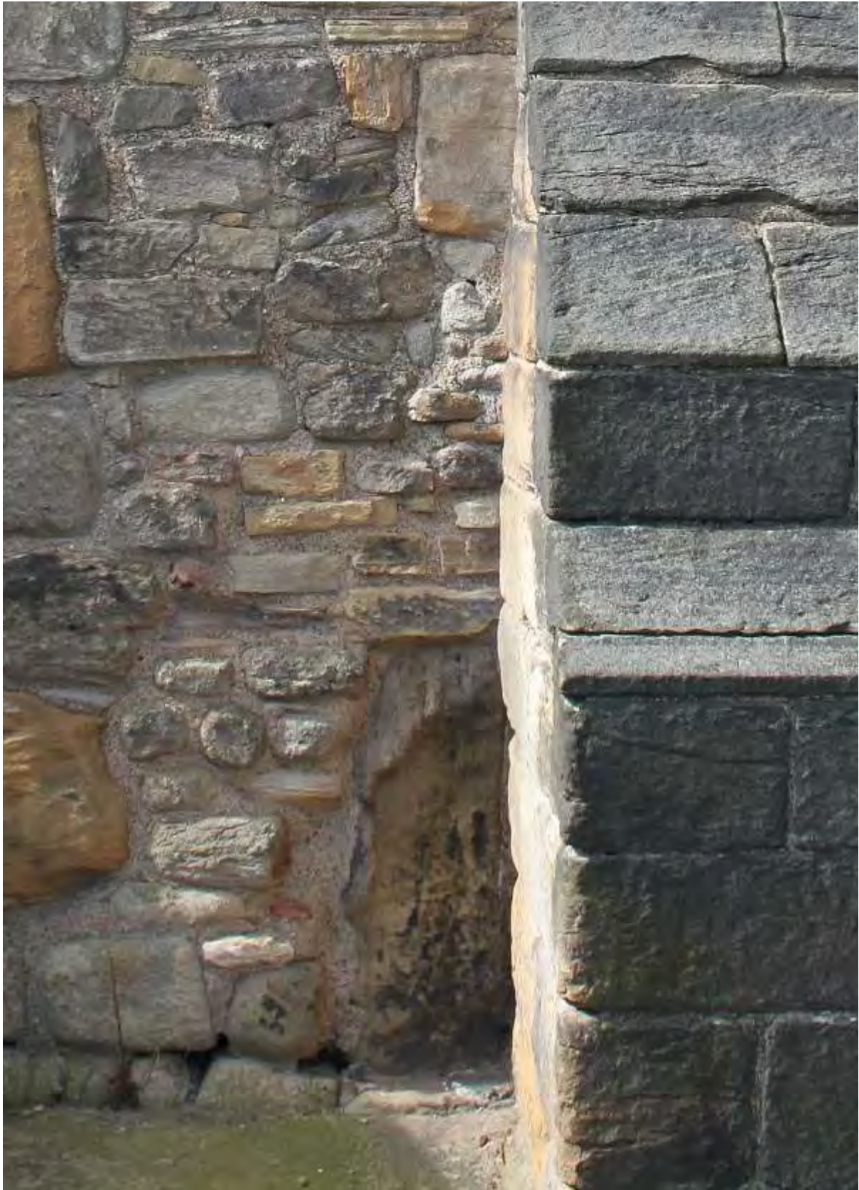
Figure 8: Detail of standing fabric visible externally at the east end of the Eastern Church. The feature is yet to be interpreted. The Type A sandstone is scorched at the base.
