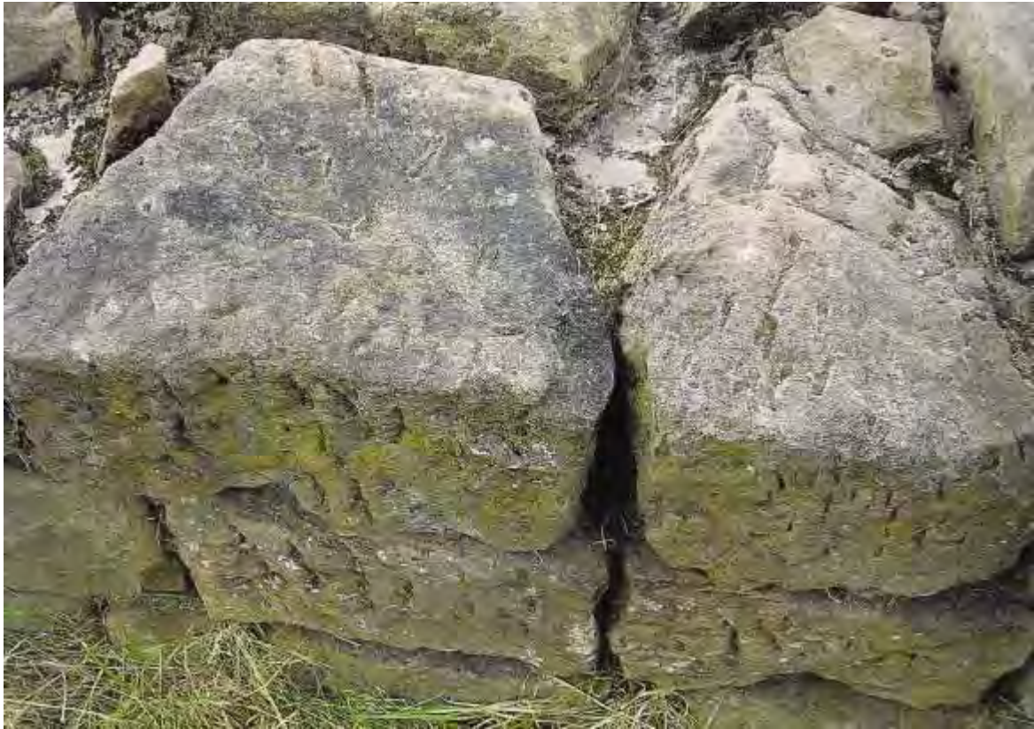
Figure 18: Arbeia: example of squared rubble blocks executed in Wrekenton Sandstone with a c. 25 cm lift height and tapered backs.
