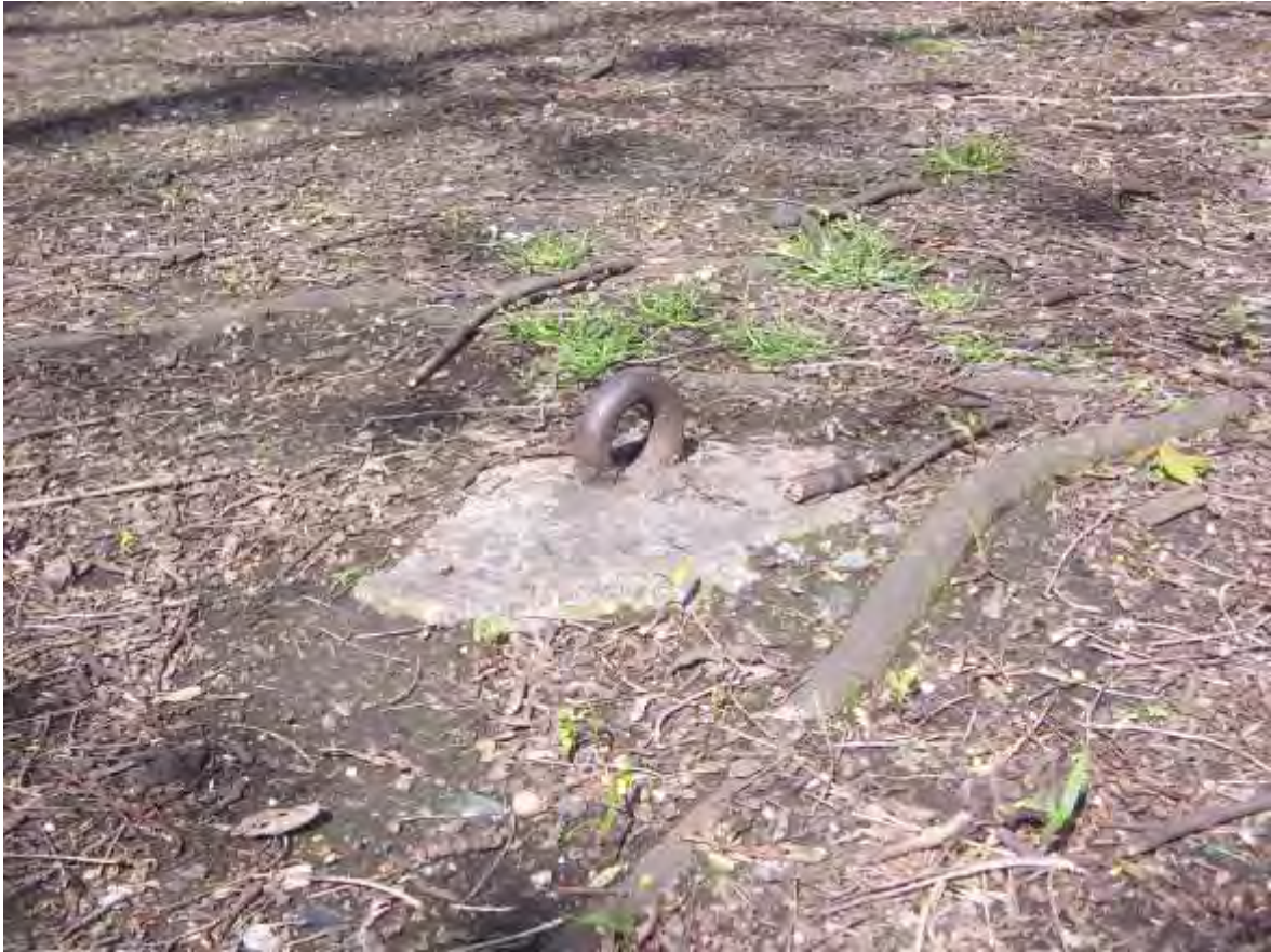
Figure 30: Example of a WWII barrage balloon tethering anchor. Results from the gradiometry indicate that a substantial part of each of these is still buried under Drewett's Park.
