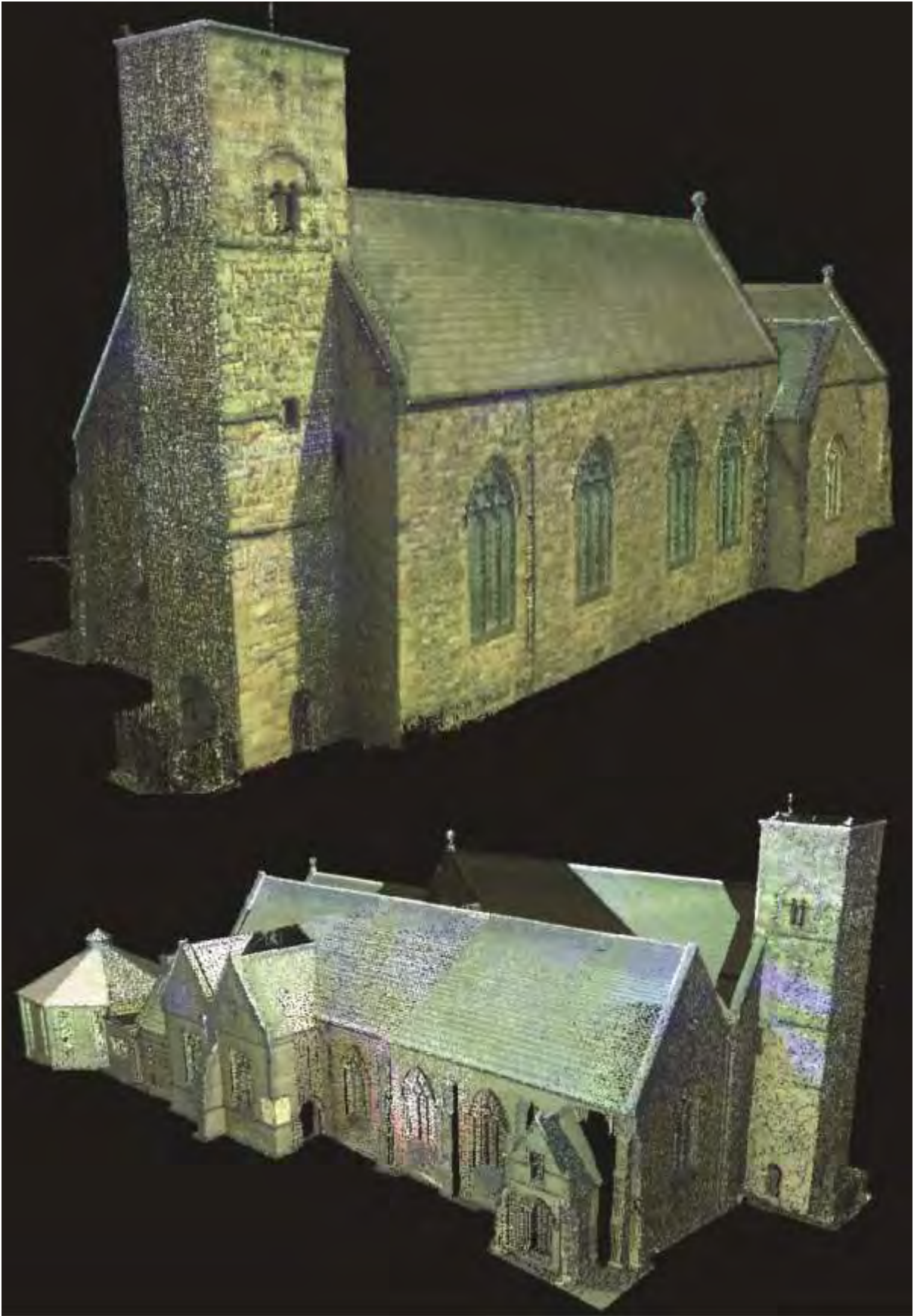
Figure 8: Point cloud for St Peter's, Weymouth viewed from west end. Opaque views using colours from camera.
